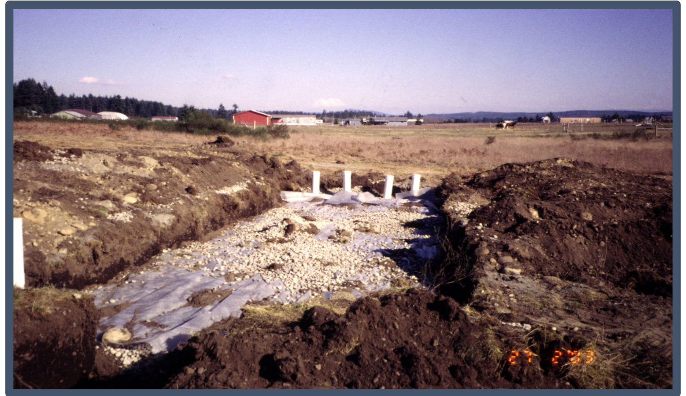
Only Shallow Rooting Plants Over Drainfield
